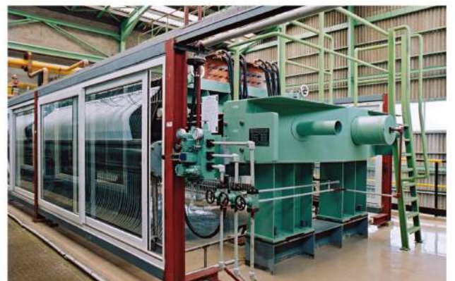
Caustic soda production facility (Source: Asahi Kasei Corporation)
