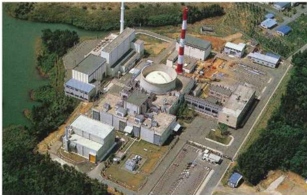
Nuclear power generation
